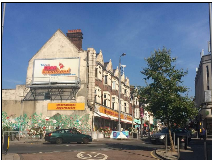
Inappropriate advertising and signage
