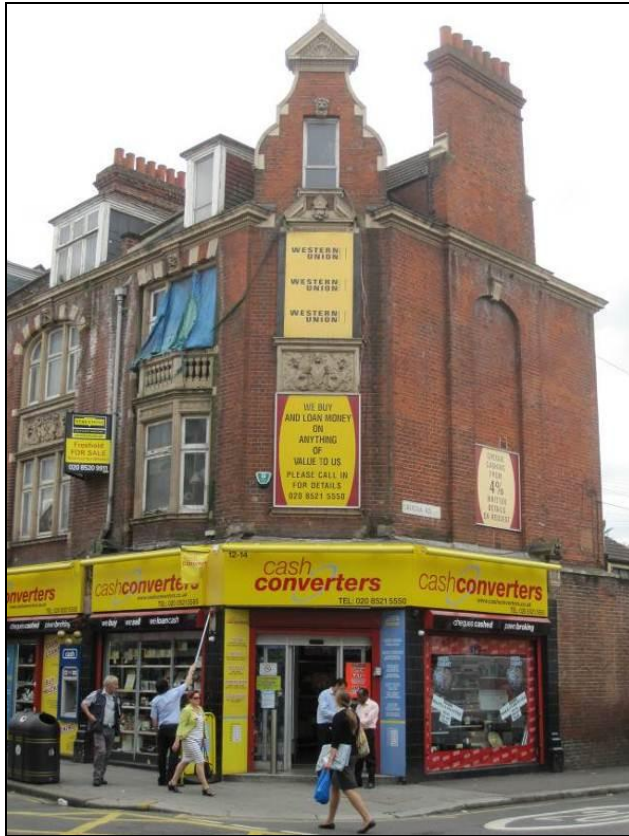
Figure 26: Large inappropriate signage in the Conservation Area
