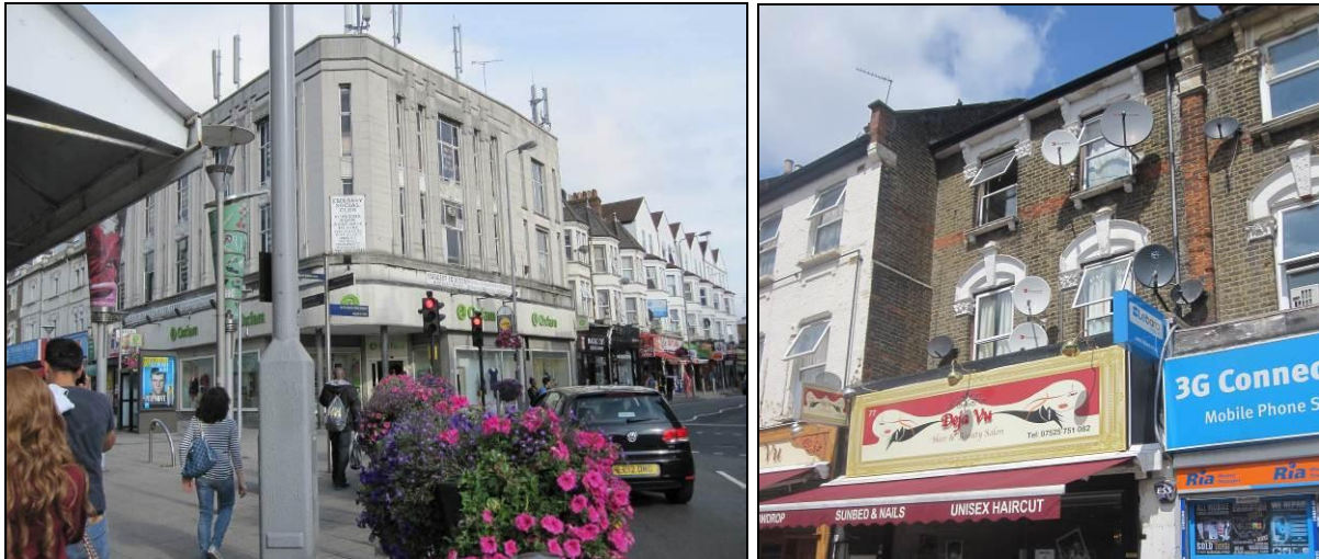
Figure 46: Phone masts above 2 High Street & proliferation of satellite dishes on northern side of High Street
