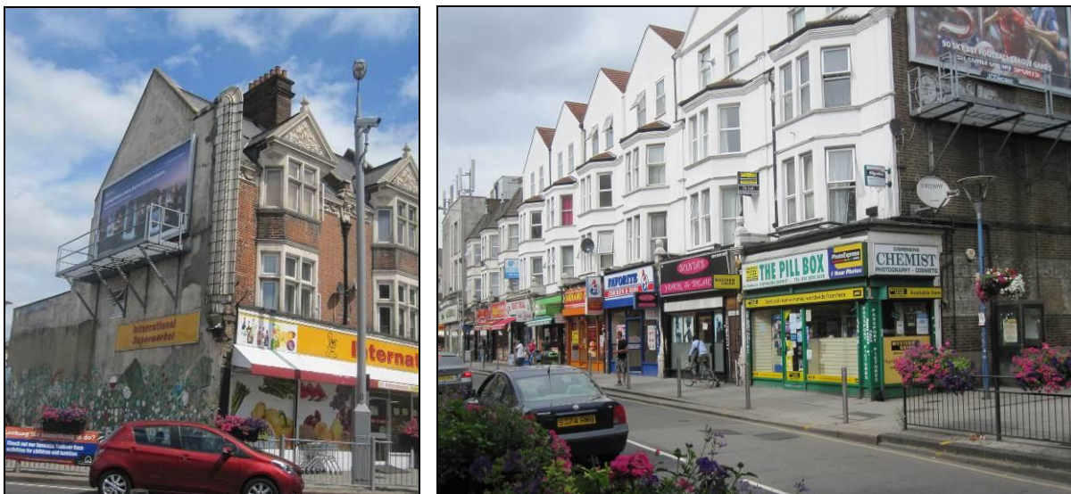
Figure 44: Large advertisement hoardings on side of building
