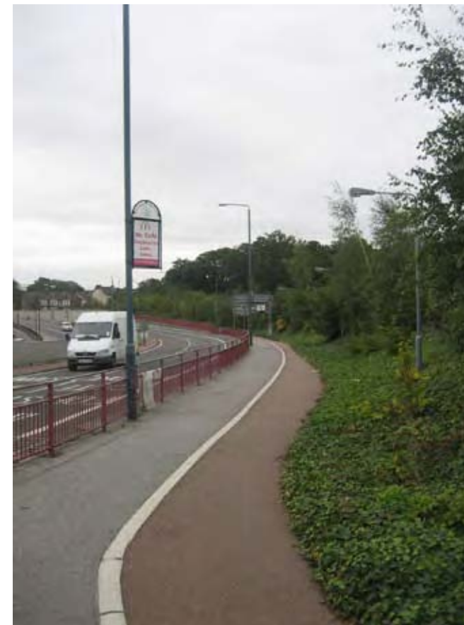
Highly engineered transition from A12 to urban environment
