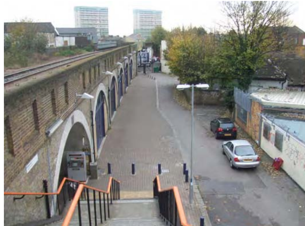
Lack of activity at interchange point
