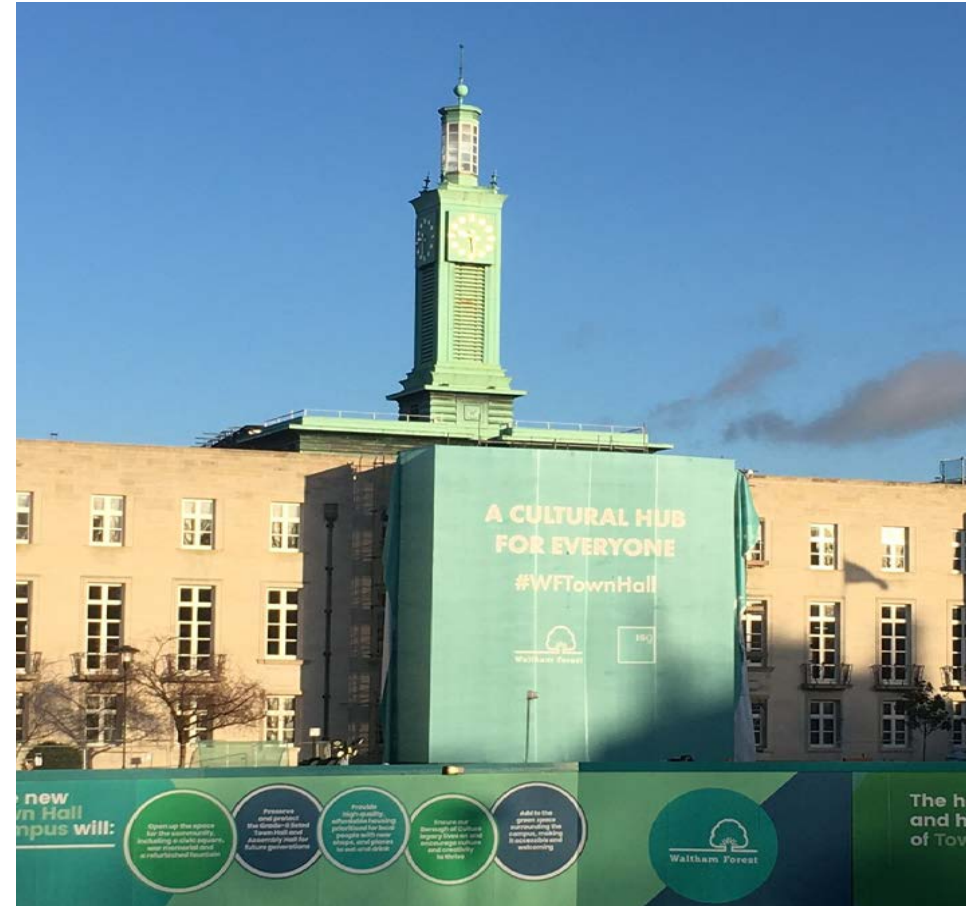
Fellowship Square Phase 1 under construction
