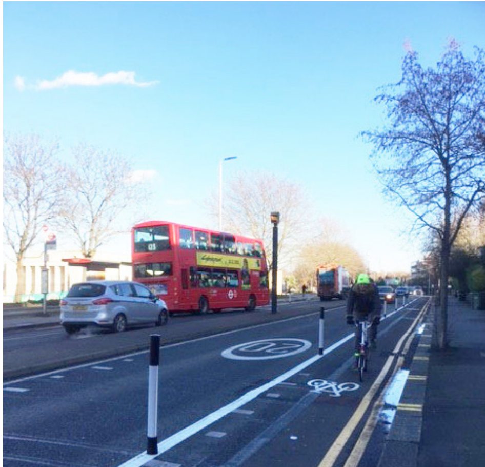
An experimental scheme recently installed provides separated cycle lanes
