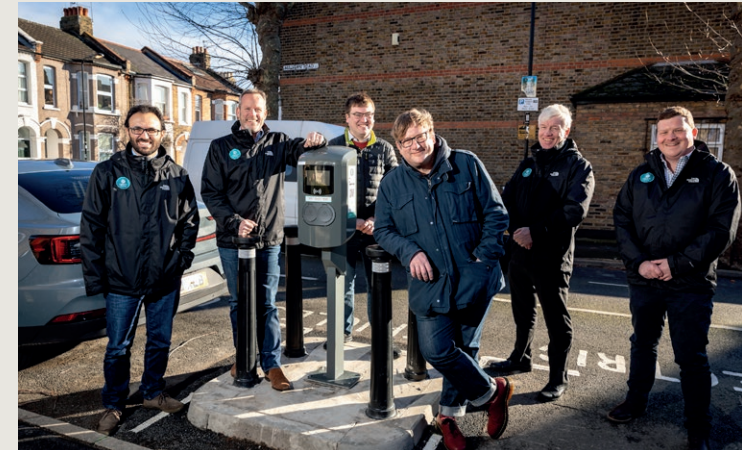
Figure 52: Electric Vehicle Charge Point on Forest Road
