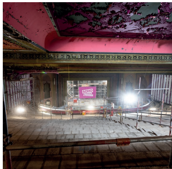
Figure 19: Construction Works in the Auditorium
