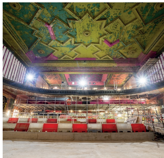
Figure 20: The Main Auditorium
