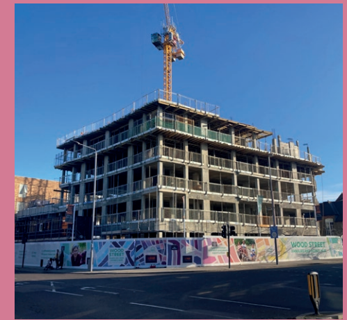
Figure 44: Families and Homes Hub Construction
