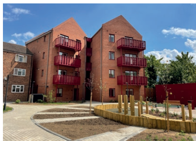
Figure 29: New Homes at Essex Close
