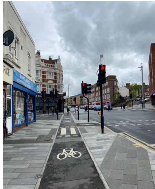
Previously Completed Works: Junction
