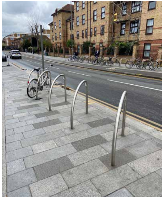
Previously Completed Works: Cycle stands
