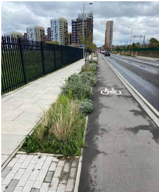
Previously Completed Works: Cycle lane and SuDs
