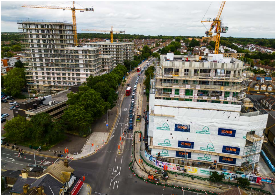
Figure 25: Construction works at the Families and Homes Hub (Sunflower House)
