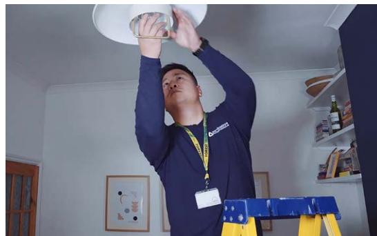
Figure 31: Domestic and communal electrical works
