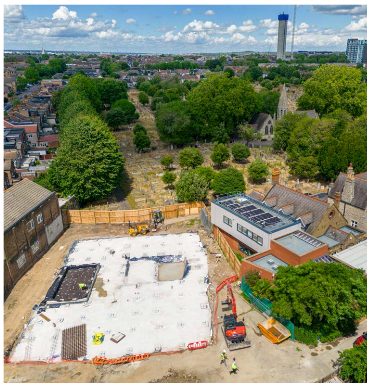
Figure 37: Construction of the new Mortuary
