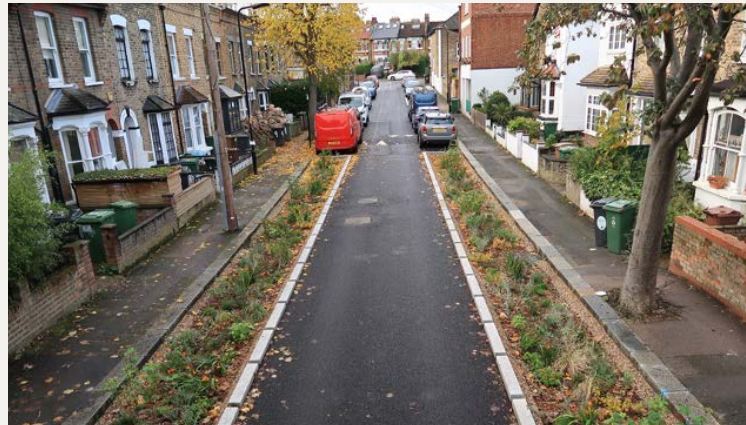
Figure 43: Upper Leytonstone Esther Road planting and flood management works completed
