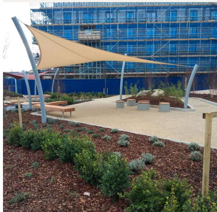
Figure 12: Construction of the new gardens at the rear of Fellowship Square
