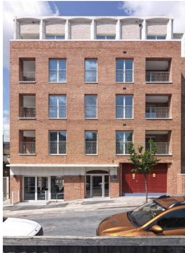
Figure 9: Finished homes at Central Parade, Walthamstow
