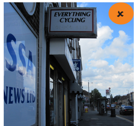
Bulky shutter housing should be avoided and where possible located behind the fascia
