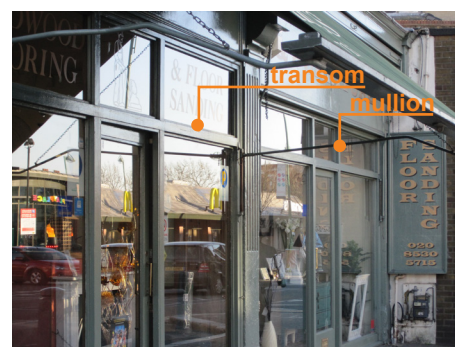
Traditional windows are divided by mullions and transoms
