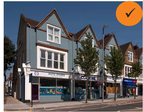
This shop extends across three units, but the fascia sign is broken into sections rather than extending across the whole shop front
