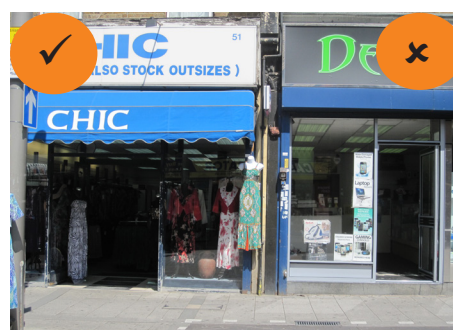
The shop to the left provides a level threshold enabling access for all
