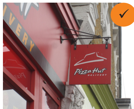
Pizza Hut's hanging sign is simple, appropriately sized and located so it does not obscure architectural details
