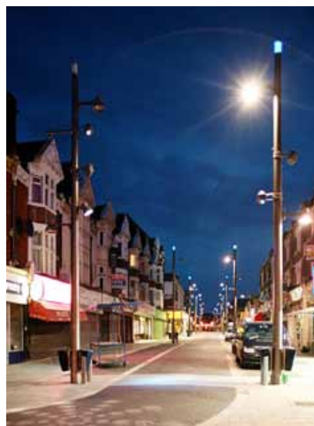
Appropriately designed street lighting
