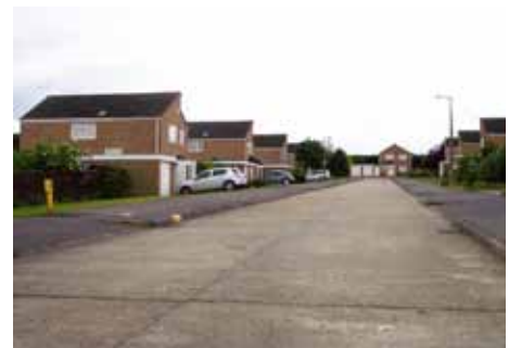
A street where the design focus has been on access and highway standards rather than as a place
