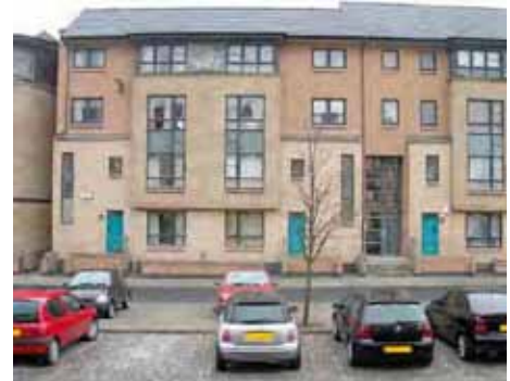
Central courtyard parking (Manual for Streets, DfT/CLG)
