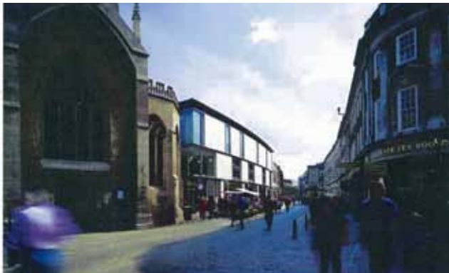
A modern retail scheme in York adjacent to contemporary buildings. The modern design has a calm low key approach, and the curve of the building and use of the stone matching the adjacent church ensures it fits well with its context (Building in Context, CABE and English Heritage)
