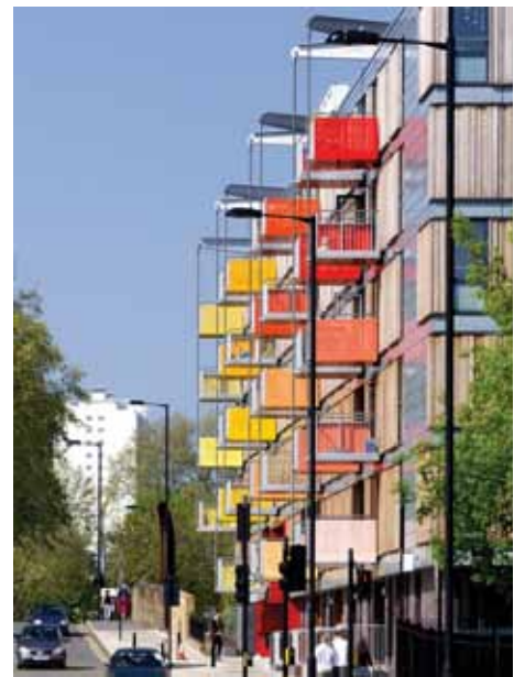
Adelaide Wharf housing scheme in Hackney shows no discernible difference between social and private housing (AHMM)
