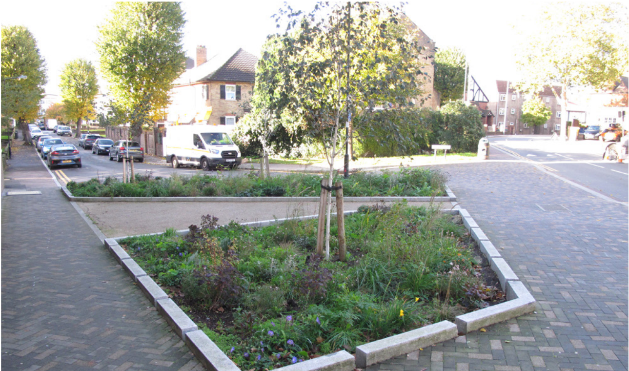
RAINGARDENS AT THE JUNCTION OF BLACKHORSE ROAD AND TENBY ROAD, E17
