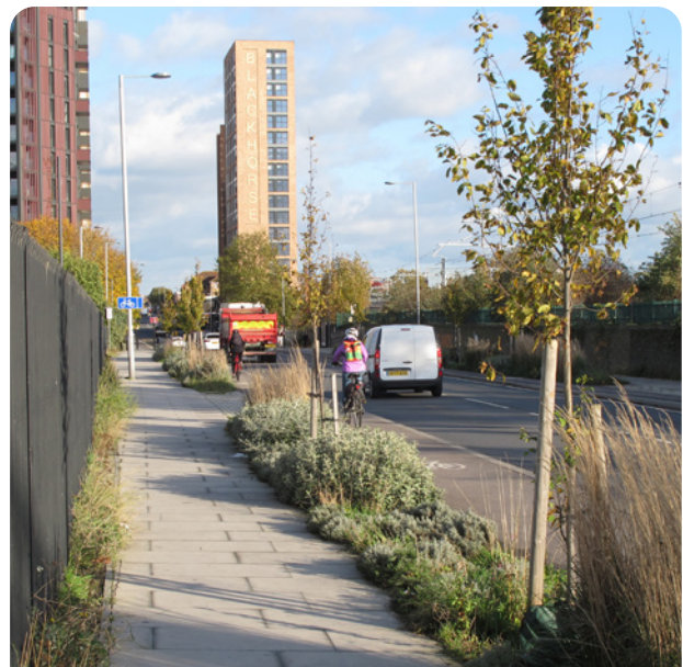
SuDS, FOOTWAY AND CYCLEWAY IMPROVEMENTS ON FOREST ROAD, E17
