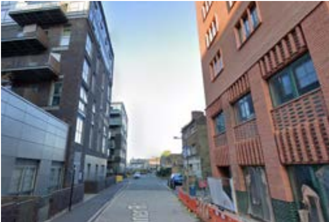
Key View 01: Brunner Road looking west
