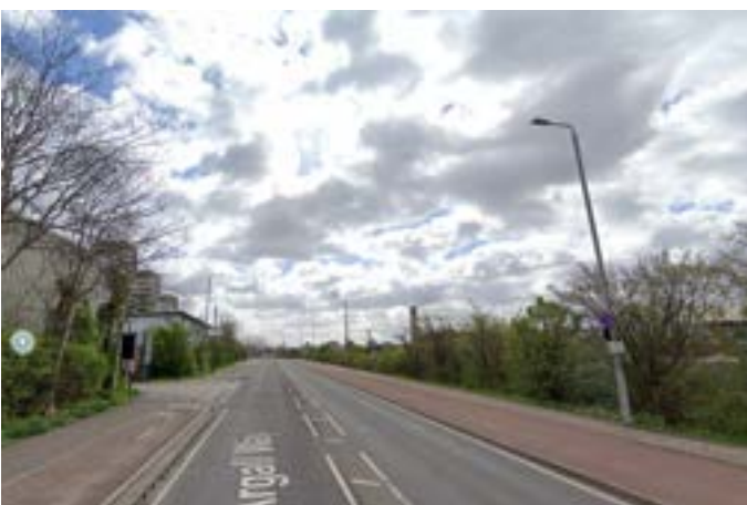
Key View 06: Orient Way looking north west
