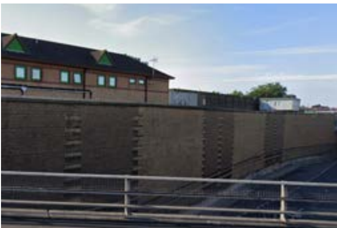
Key View 09: A106 looking south
