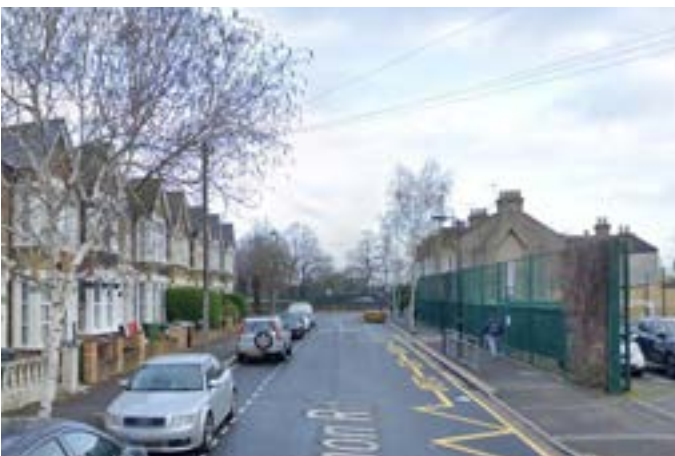
Key View 03: Vernon Road looking north west
