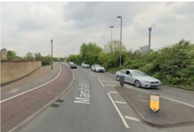
Key View 08: Marshall Road looking south east
