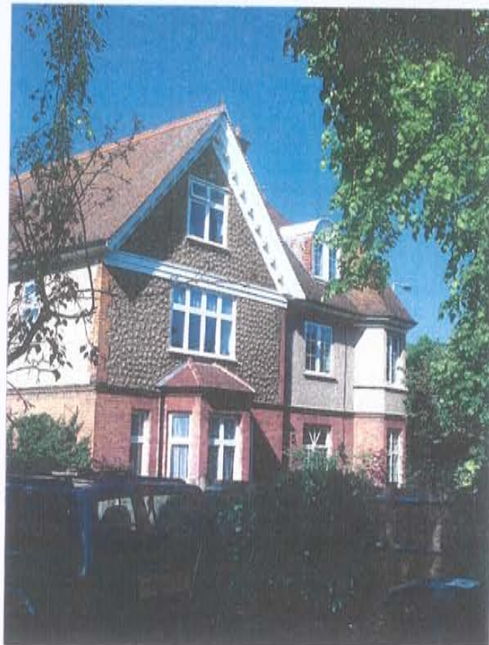
Some examples of the spacious detached and semi detached houses erected during the early period of suburbanisation following the arrival of the railway and World War I, featuring clay tiled roofs, roughcast render, timber windows & orange/red bricks.
