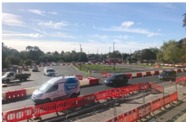
Progress on Whipps Cross Junction
