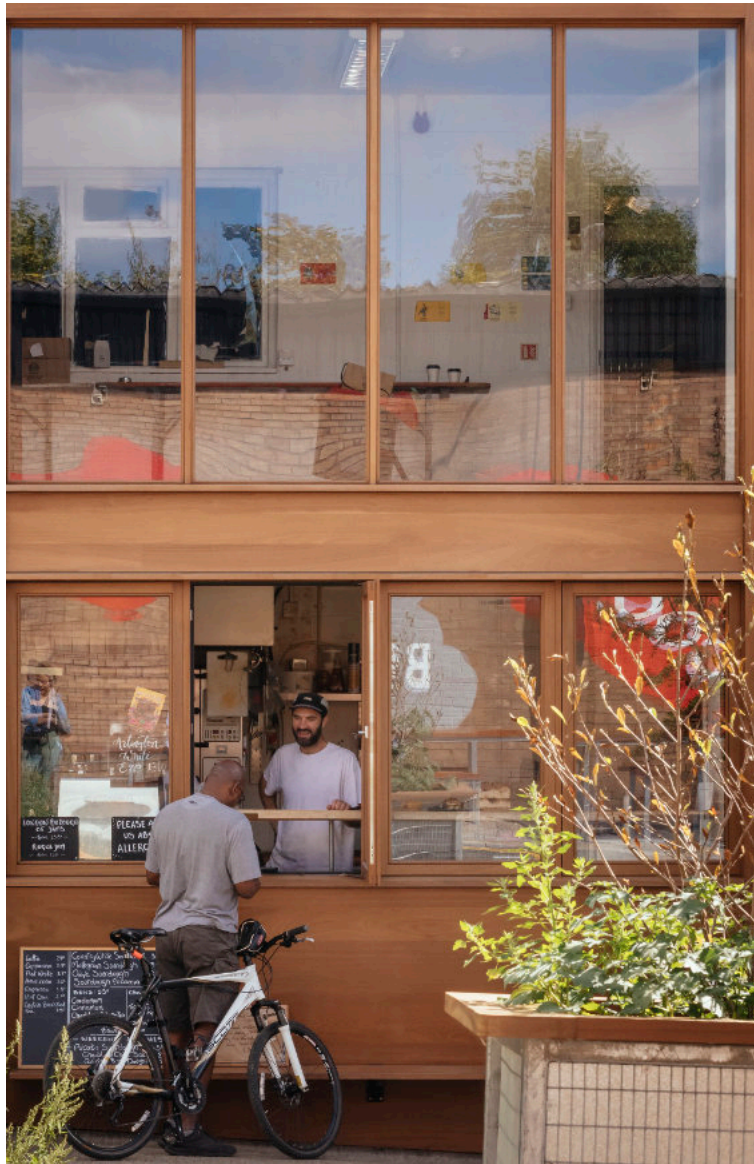
Lockwood Way, We Made That © Jim Stephenson
