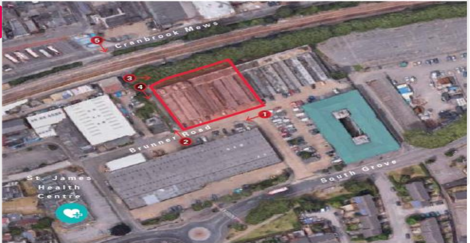
Aerial view from the south, site highlighted in red
